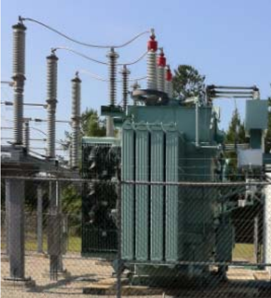
Two Winding Three Phase Transformer
